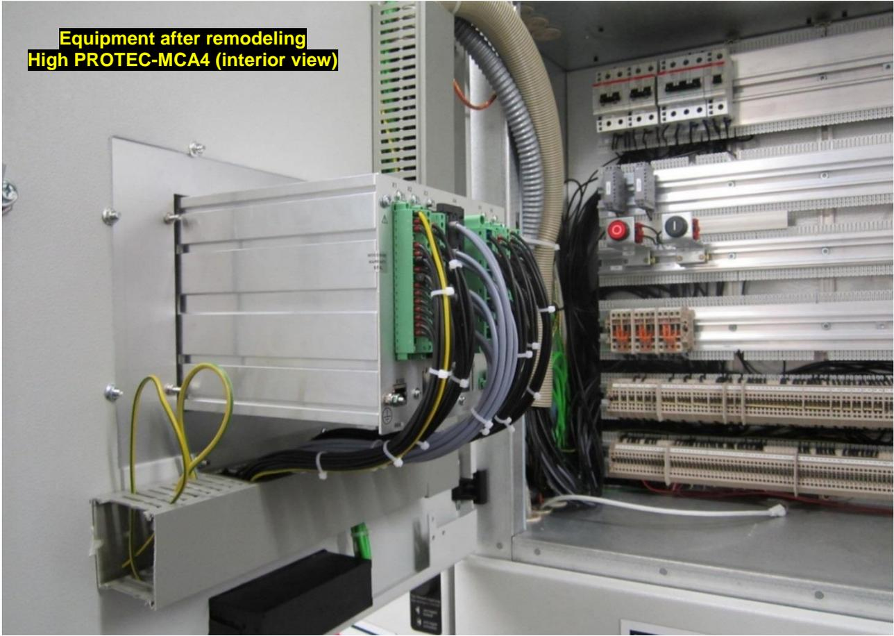
**Equipment after remodeling to HighPROTEC-MCA4 (interior view)**
